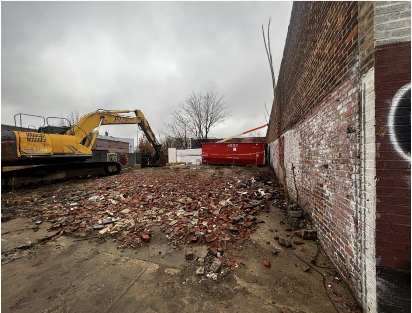
Current construction site at 447 Wales Avenue, courtesy of Civic Builders
